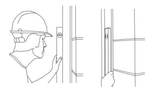
3. Ensure the frame is vertical in both planes, particularly the hinge jamb.
